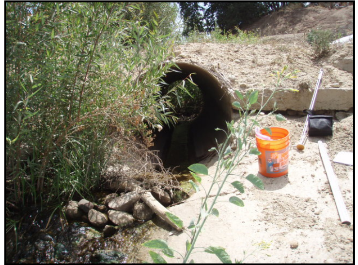
View upstream (toward the S) toward the sample site at the culvert outfall.
