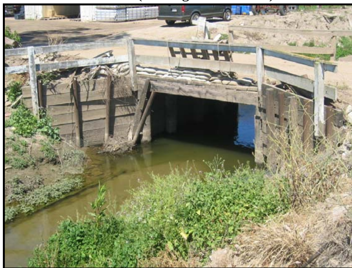
View toward the NE (looking downstream)
