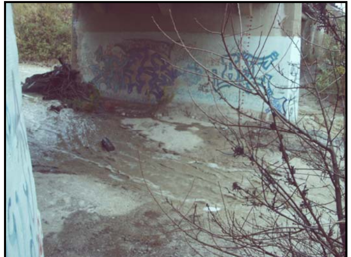
View from W bank looking NE (upstream) at the bridge pier.
