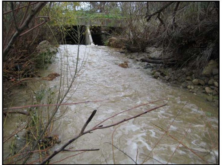
View from sampling location downstream toward the Hwy 126 Bridge.
